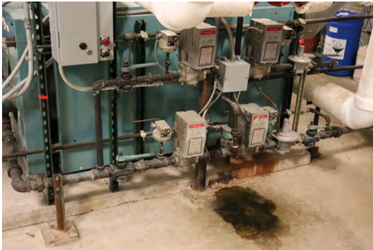
Mechanical heating system upgrades
