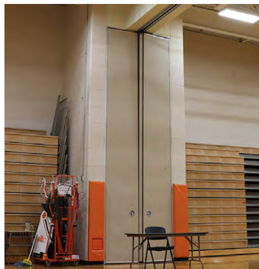
Gym partition upgrade
