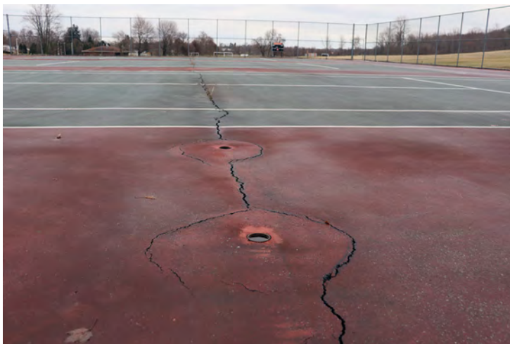
Tennis court restoration
