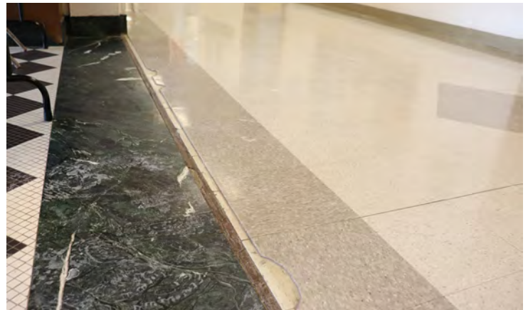
Main High School corridor interior finish improvements
