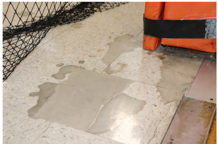
Gymnasium floor restoration
