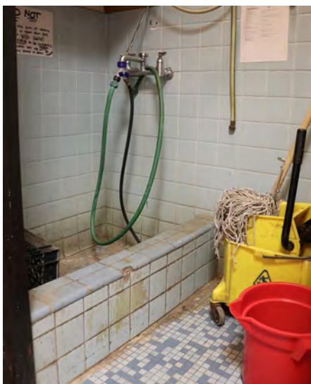
Service area plumbing and interior finish improvements
