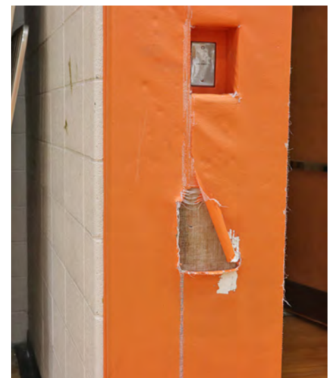
Gymnasium wall pad replacement
