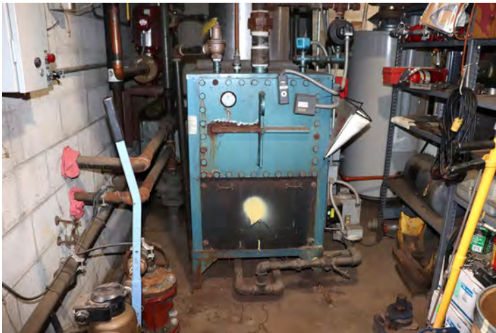
Transportation facility heating upgrade
